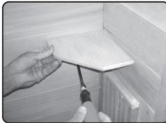
Attach cup holders in the fore left corner and the fore right corner (when sitting in the sauna).
