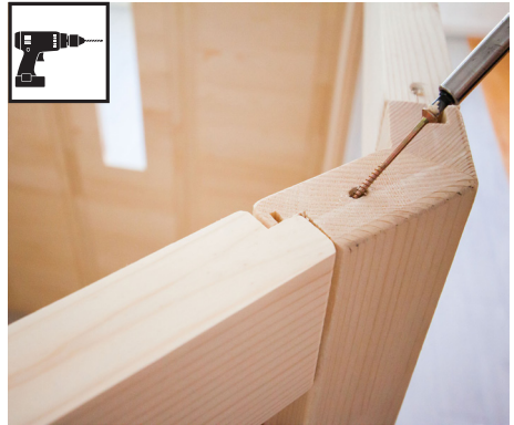
3 mm drill bit, 1 screw 4 x 70 mm
