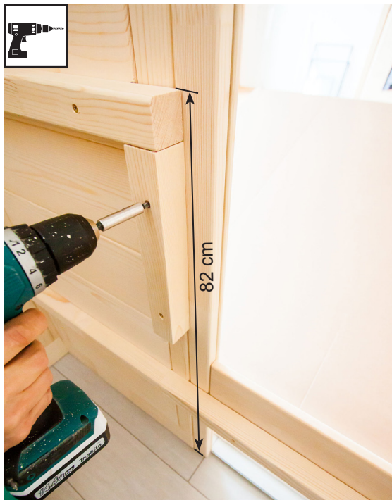
3 screws 5 x 70 mm 2 screws 4 x 60 mm
